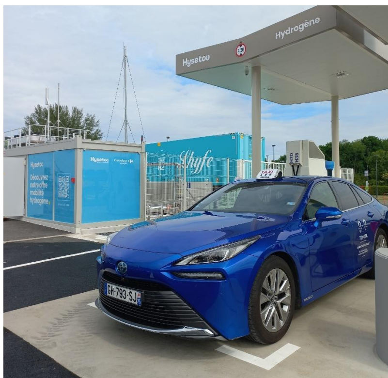
Caption: Hydrogen station of the HysetCo network, in Collégien (77), powered by green and renewable hydrogen from Lhyfe (container in the background). HD visual on this link . Credit: HysetCo and Lhyfe.
