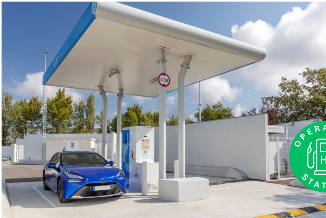
First HRS station installed in Saint-Priest in late 2021
